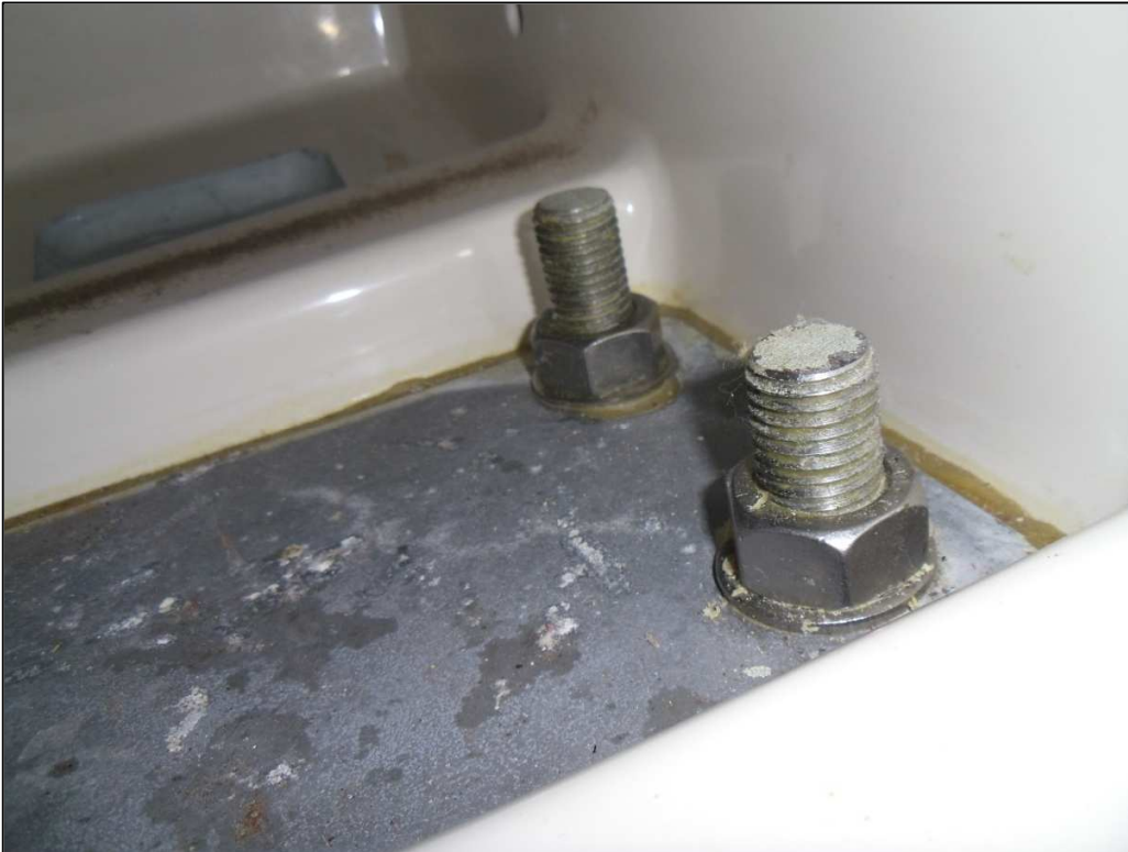
Fig.2 – section of keel bolts showing their condition which is the same for all.
