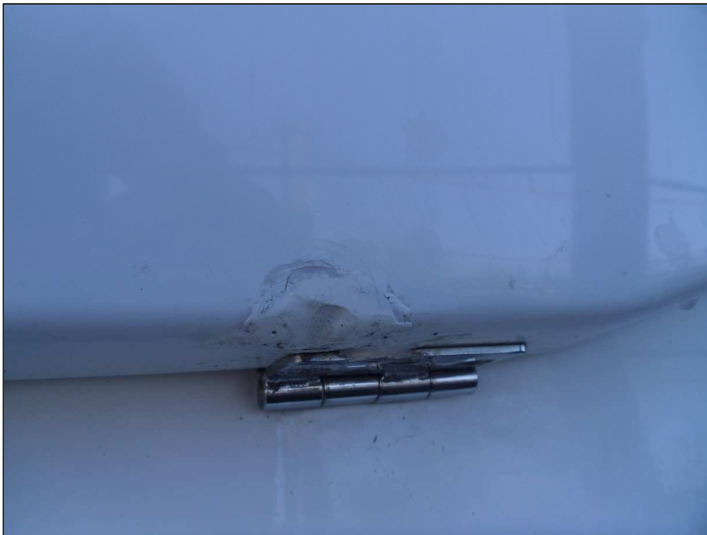
Fig.1 – damage to platform starboard hinge plate and surrounding gelcoat.
