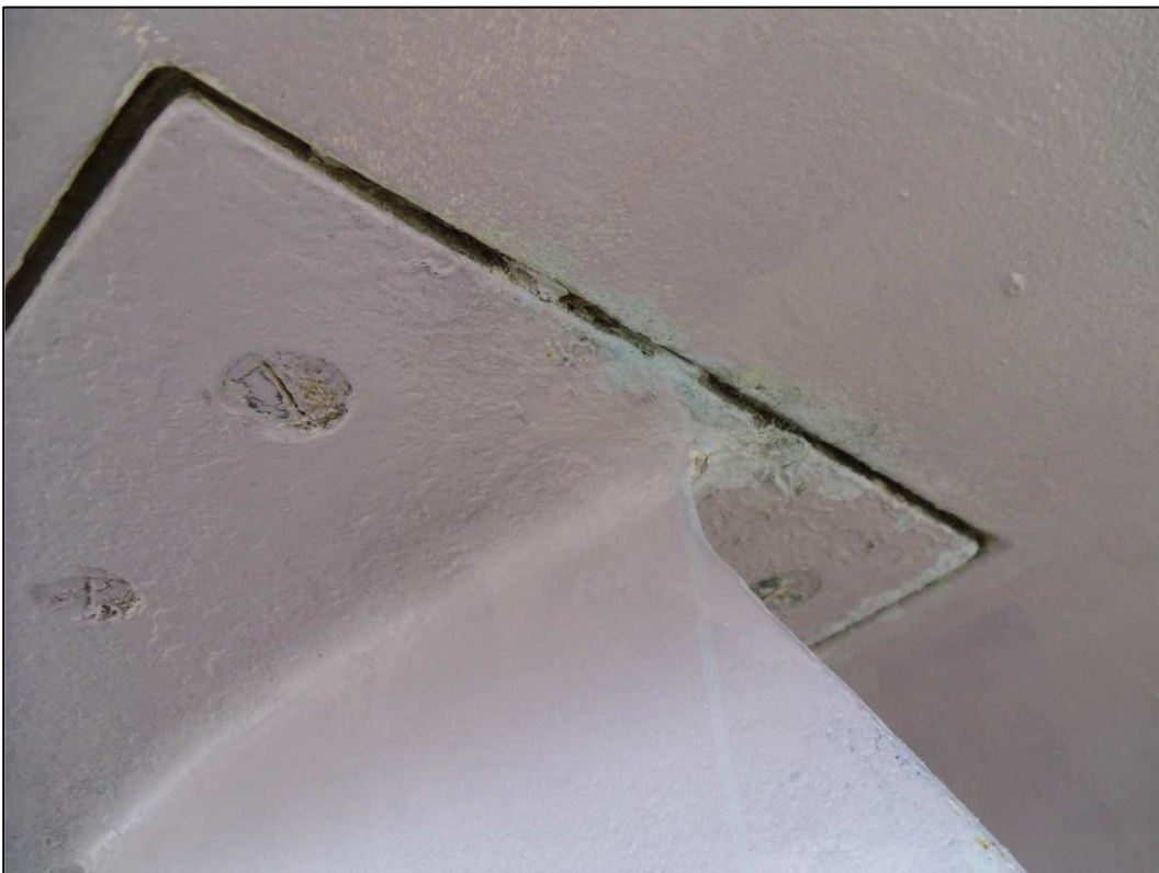
Fig.3 – some light weeping / deposits from the aft end of the port palm.
