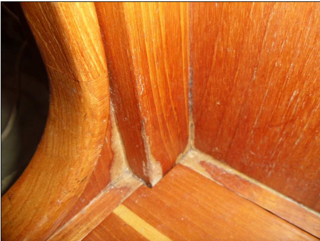
Fig.2 – areas of water staining at the base of the compression post.
