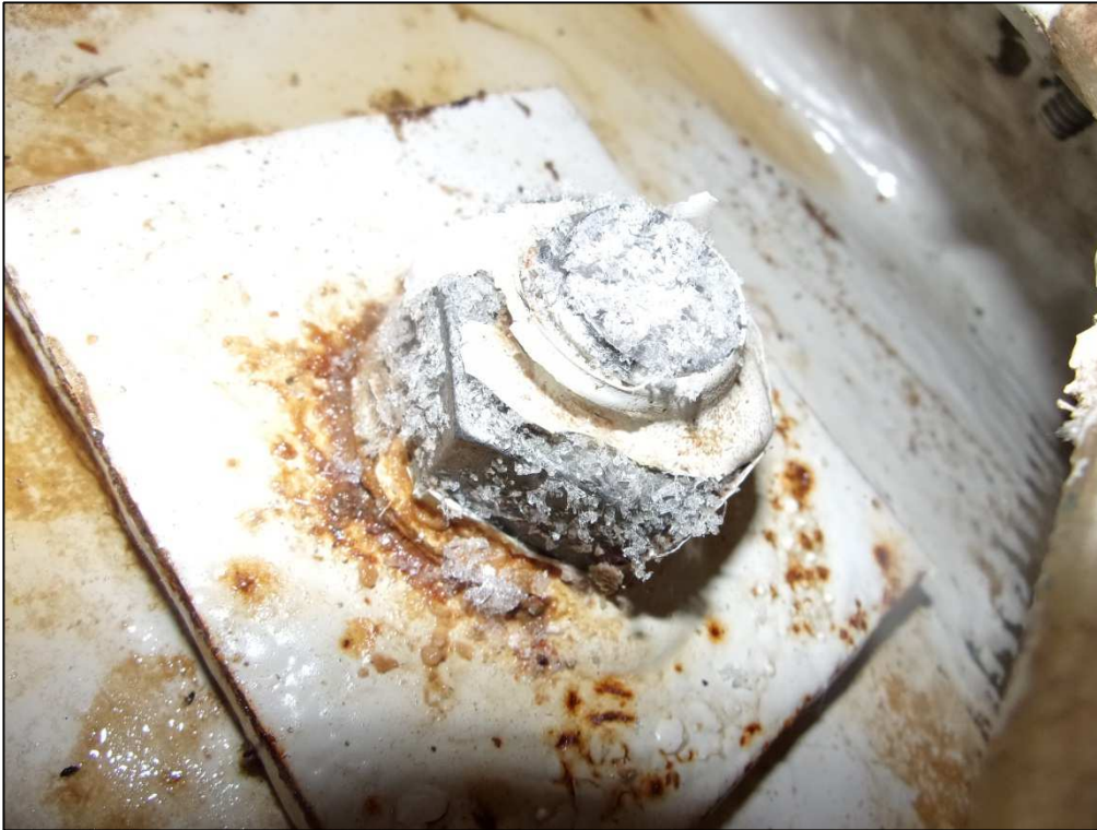
Fig.1 – keel bolt and securing plate showing surface corrosion.
